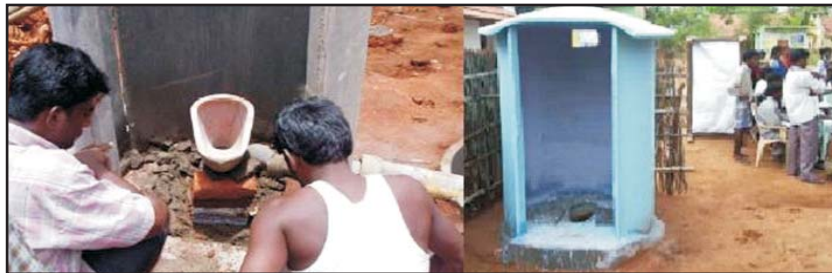
Students of Diploma in Sanitation Inspector course building demonstration latrines in village
